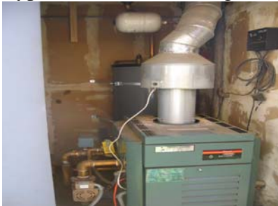
Typical boiler with storage tank
